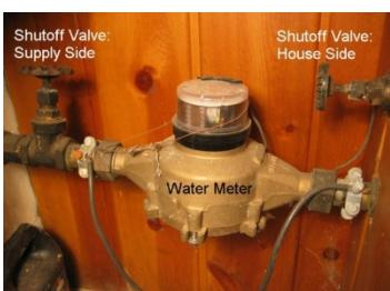
Locate the pipe that runs from the water meter to your house. Wrap a piece of string around the pipe, mark it, then measure how much string it took to go around the pipe. Identify the size and type according to the chart below.
