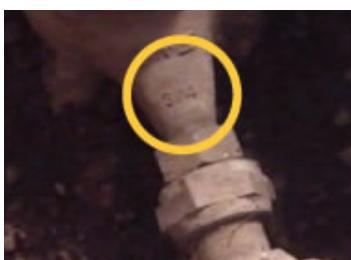
The meter size ( 5/8", 3/4" or 1") is usually stamped on the outside of the meter.
